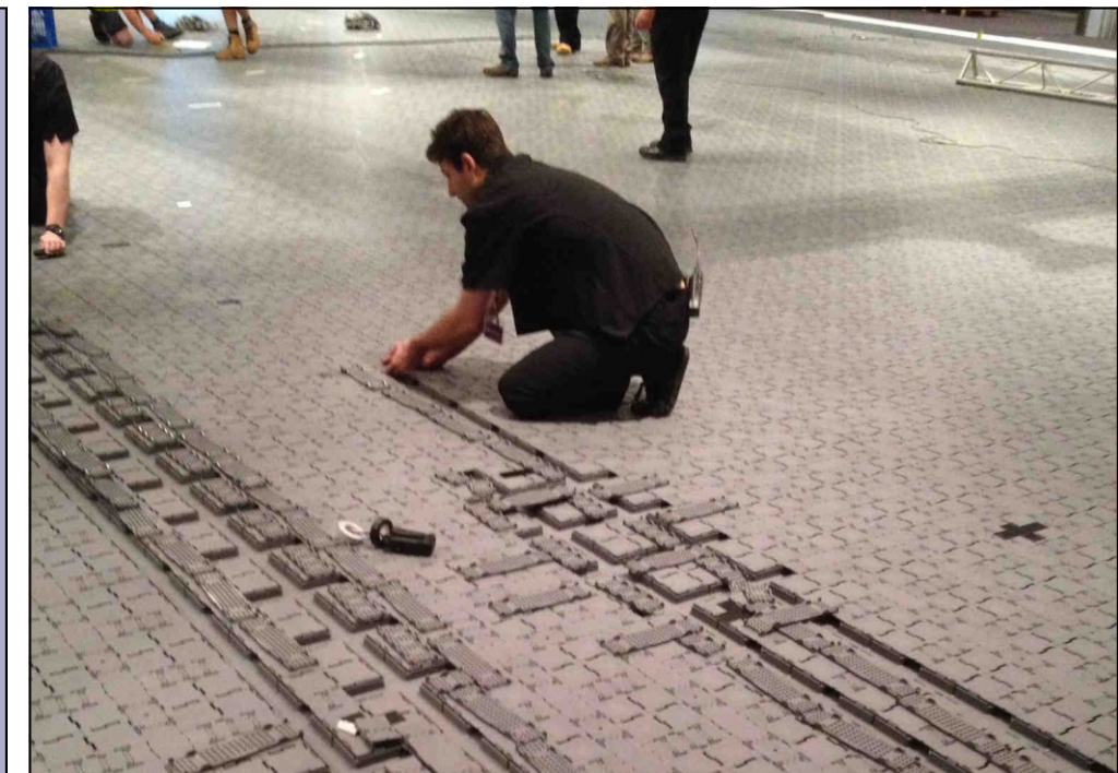
Access to cable channels is simple and straight forward
